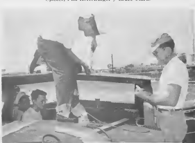
LENDING A hand on construction, Mate Bill Myers, right, works with Bruce Clark, Frank Barnes and Phil Heffelfinger.
